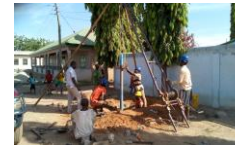
Manual Drilling Crew
