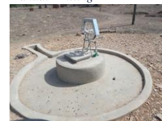
Rehabilitated hand dug well
