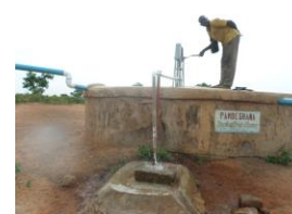
40,000 liters rain water tank
